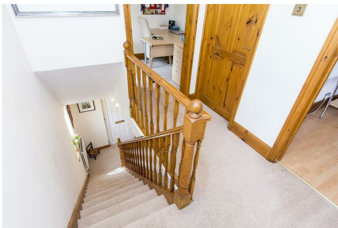
Double-glazed window to side elevation. Timber balustrade. Access to loft space. Pine doors to rooms.
